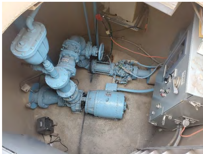
Figure 3-14 McNary Booster Pump
