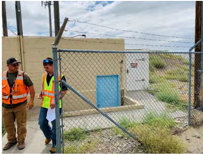
Figure 3-1 McFarland Well Pump House
