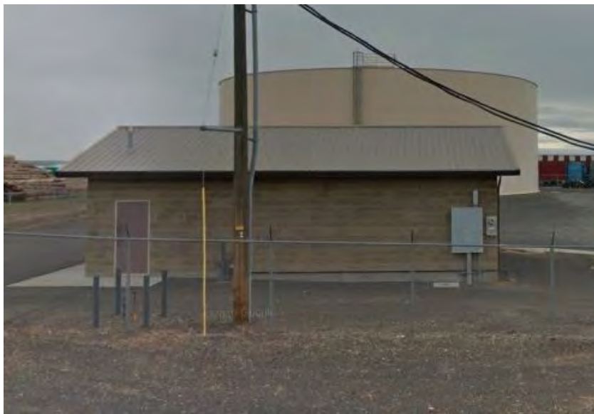
Figure 3-15 Golf Course Booster Station
