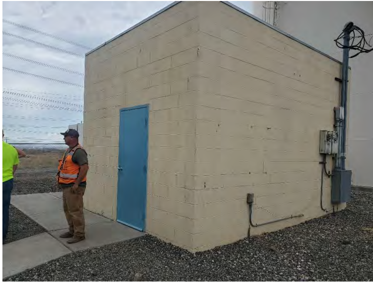
Figure 3-3 Intertie Well Pump House
