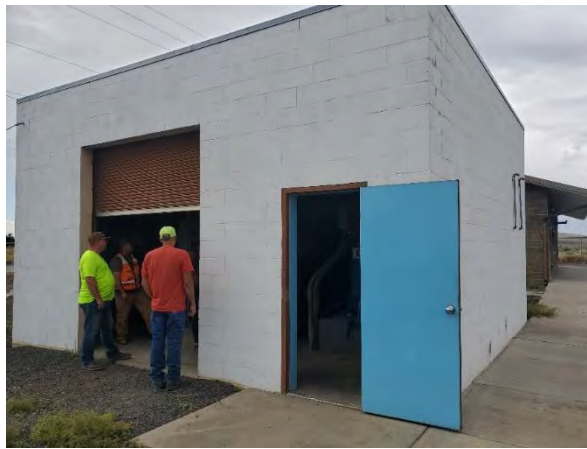
Figure 3-5 Golf Course Well Pump House
