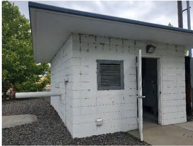
Figure 3-7 Port Well Pump House
