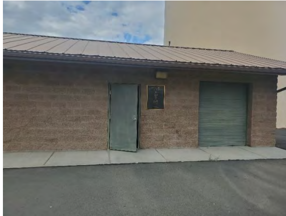
Figure 3-11 Coyote Booster Station
