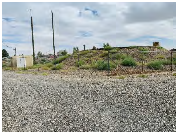
Figure 3-18 McFarland Concrete Reservoir
