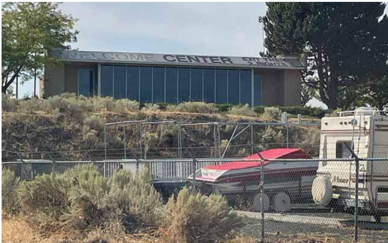
LANDMARK.1 LETTERS/GRAPHIC/SIGN on top of Welcome Center (Visible from Bridge)
