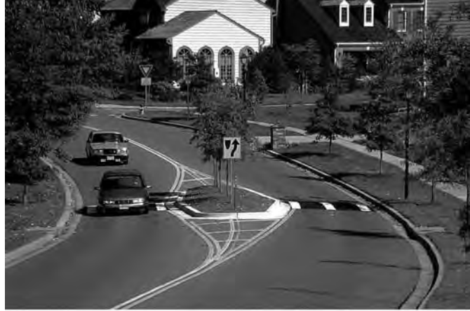
Refuge island with speed hump.
