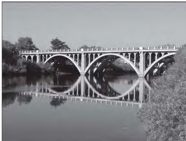
Umatilla Bridge from fishing platform on River Trail.
